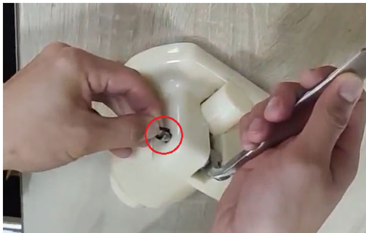
1. Remove Stem O-ring
