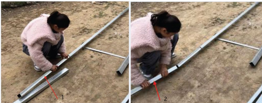
1- Connect the small tube section
