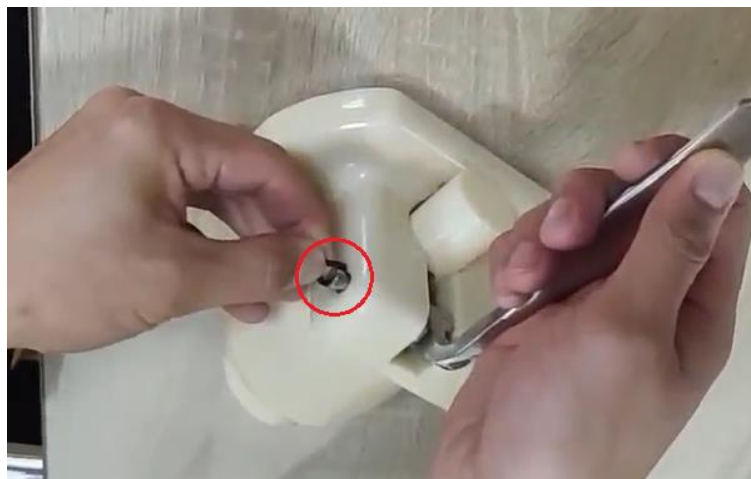
1. Remove Stem O-ring
